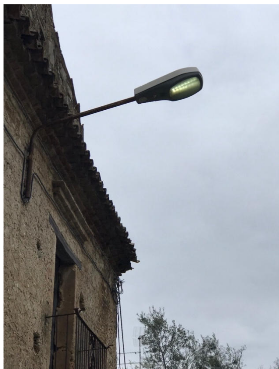
FOTO 3. - Armatura STRD Led B.M. 1
