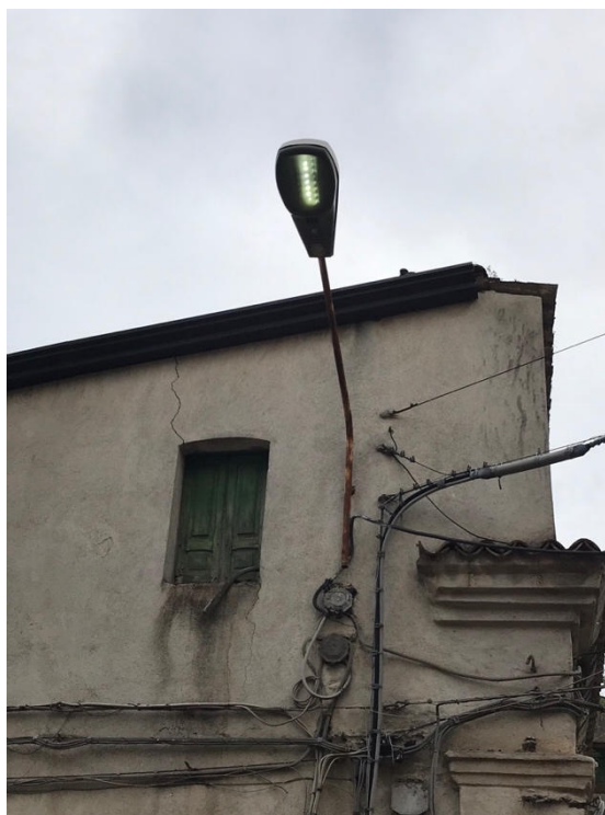
FOTO 10. – Armatura stradale LED B.M. 1
